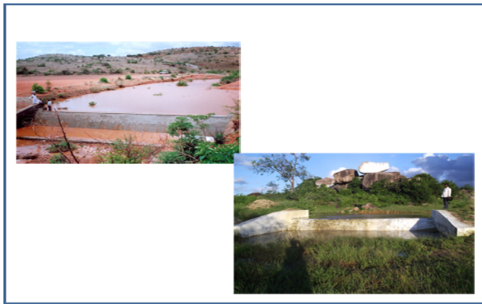
Check Dams in large open areas and on first or second order streams
